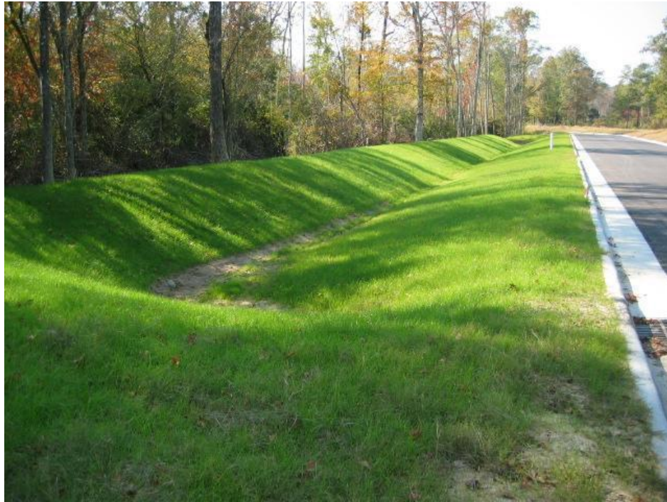
Grassed Swale. Photo Courtesy of: Thomas Engineering, PA. http://www.thomasengineeringpa.com/photo_gallery/photo_gallery.htm
