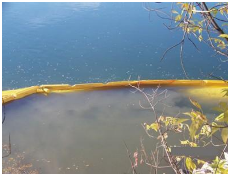
Floating turbidity barrier. Photo courtesy of Terra Erosion Control Ltd.
