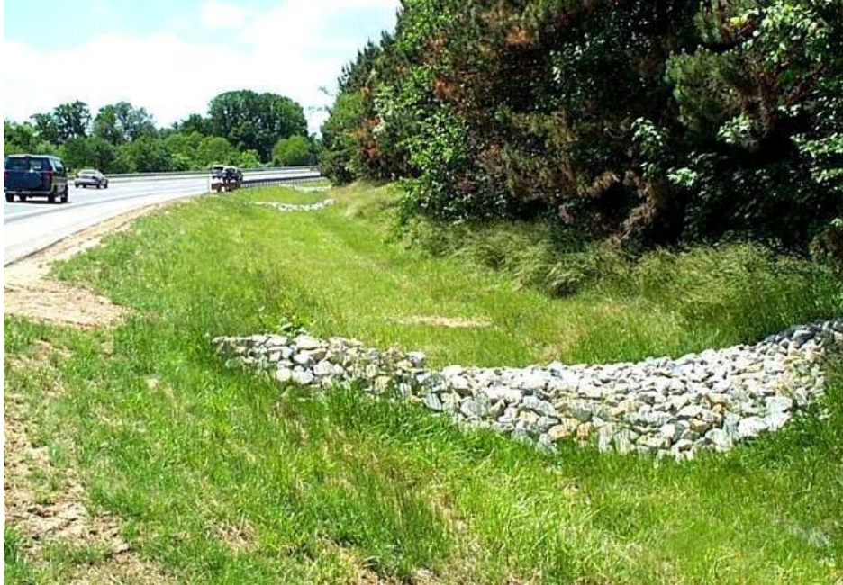
Waterway drop structure. Source: State of Delaware DOT
