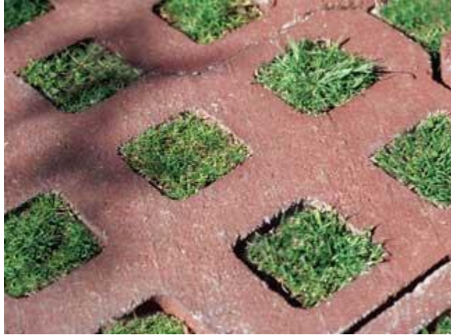
Figure Grid Pavements. Photos courtesy of: www.soilretention.com
