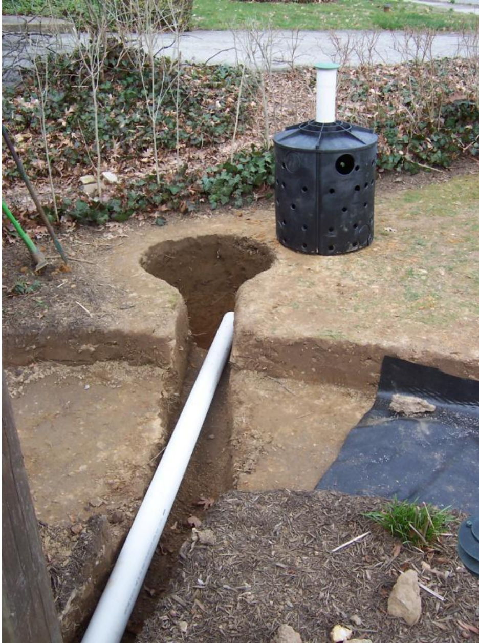
Dry well being installed. Photo courtesy of Canela Landscaping. http://www.canalelandscaping.com
